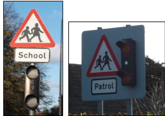
Wig-wag lights can be mounted below the sign assembly or at the side usually as part of a backing board.
